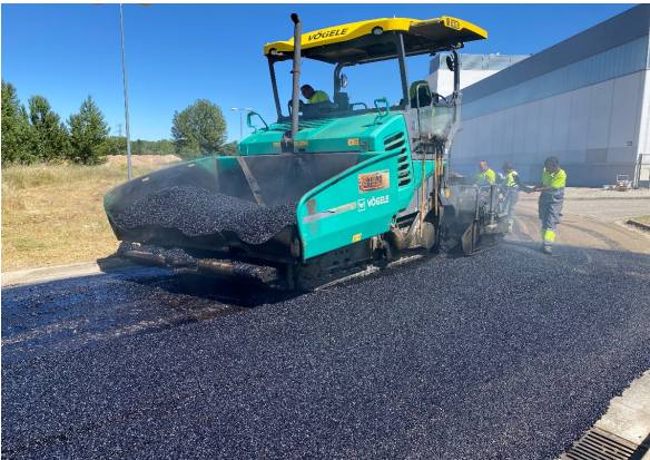
Figure 5 and 6. Bituminous mixtures manufactured with steelmaking slags
