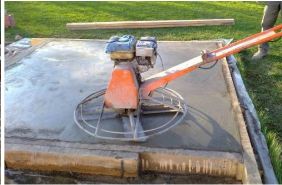
Figure 3 and 4. Concrete pavements manufactured with steelmaking slags
