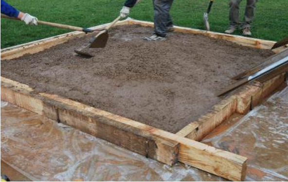
Figure 3 and 4. Concrete pavements manufactured with steelmaking slags
