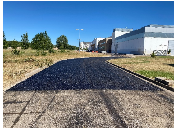
Figure 5 and 6. Bituminous mixtures manufactured with steelmaking slags
